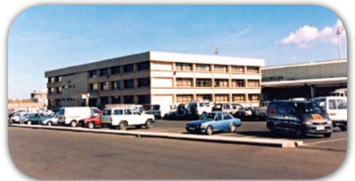
The New Cargo Terminal facility.
