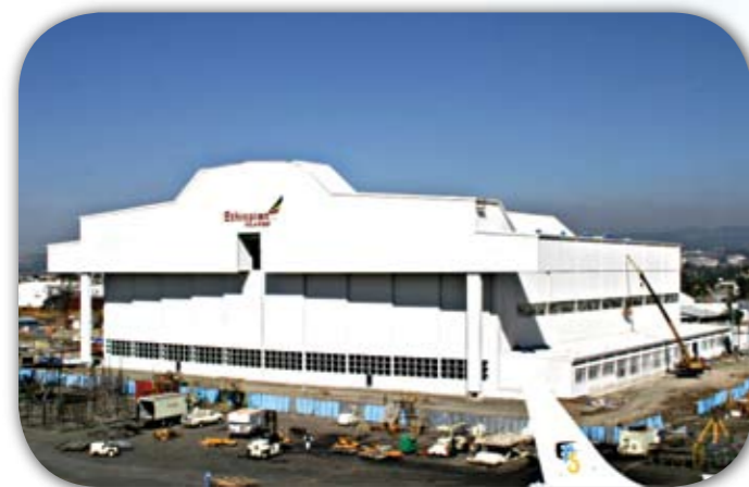
The New Maintenance Hangar.
